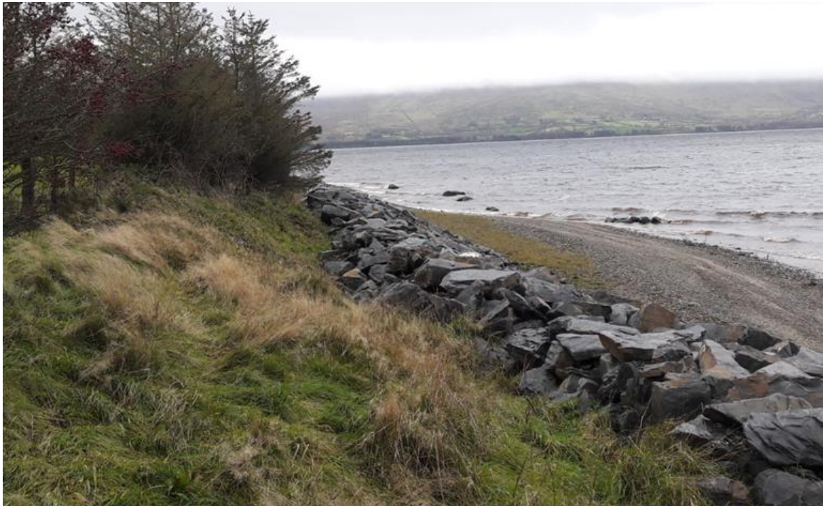
Figure 7 Existing Rock Armour at Lacken
