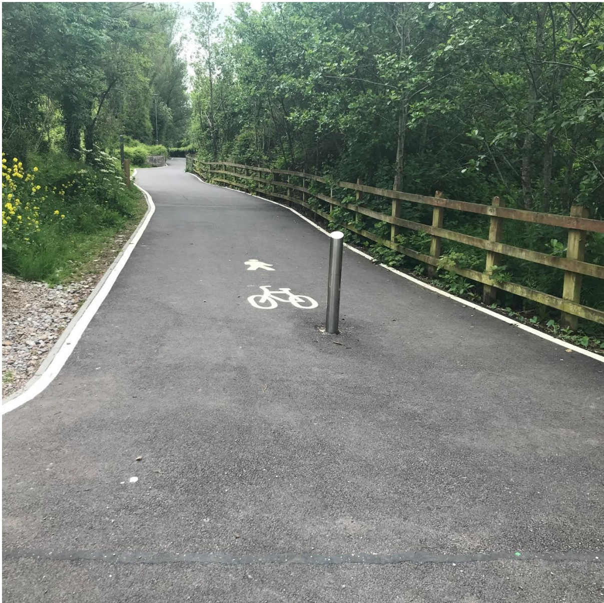
Figure 5 Bollard Access Control
